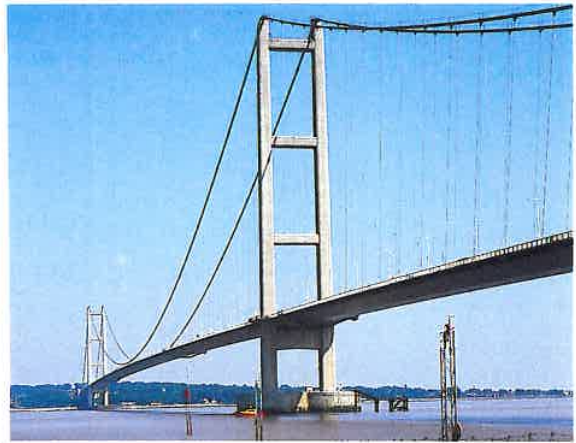
Suspension bridges are usually erected when very long spans are involved or when the soil is too unstable to support the piers. One of the longest
