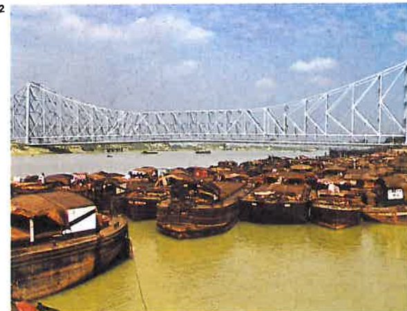
2 The Howrah Bridge in Calcutta is a typical steel truss cantilever bridge spanning a distance of 453m. The two main piers of this
