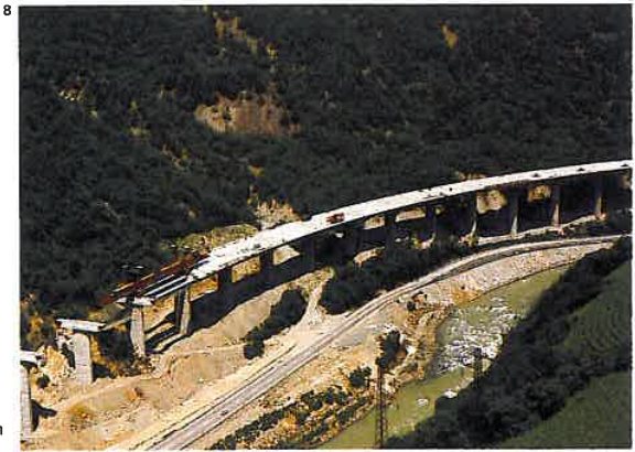
5 Motorway interchanges are designed to allow the free flow of traffic without intersections and this involves the use of a lot of bridges together with elevated viaducts. Most of these bridges are of the simple beam type and reinforced concrete construction is widely used, either as prefabricated sections or cast in position. When motorways are constructed, bridges have to be built before roads.
