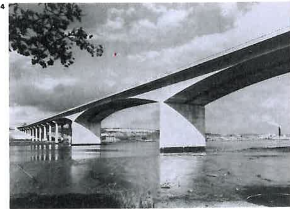
3 The Gladesville Bridge over the Parramatta River at Sydney, Australia, is a 305m span concrete arch with a height of 41m. It was formed from pre-cast elements erected on a steel centring.
